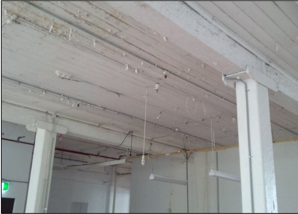
PHOTO 3: GROUND FLOOR COLUMN, BEAM AND CEILING CONSTRUCTION
