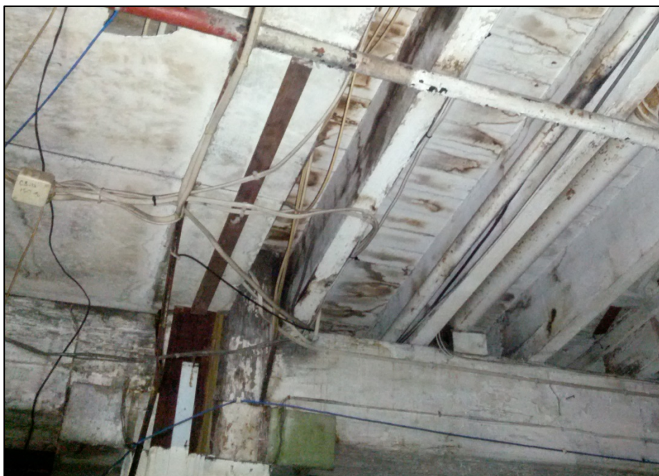
PHOTO 2: GROUND FLOOR JOISTS AND FLOORBOARDS
