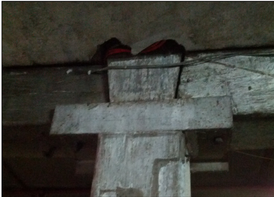
PHOTO 1: BASEMENT COLUMN TO BEAM CONNECTION
